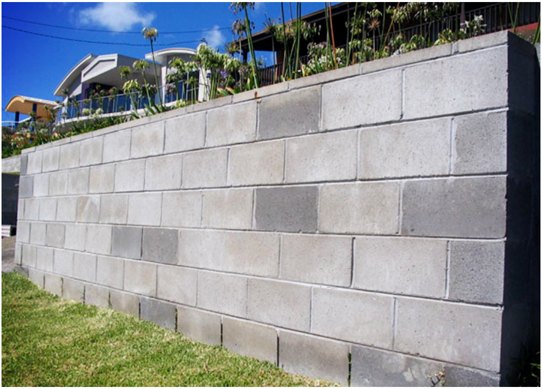
CONCRETE BLOCK RETAINING WALL IMAGE
